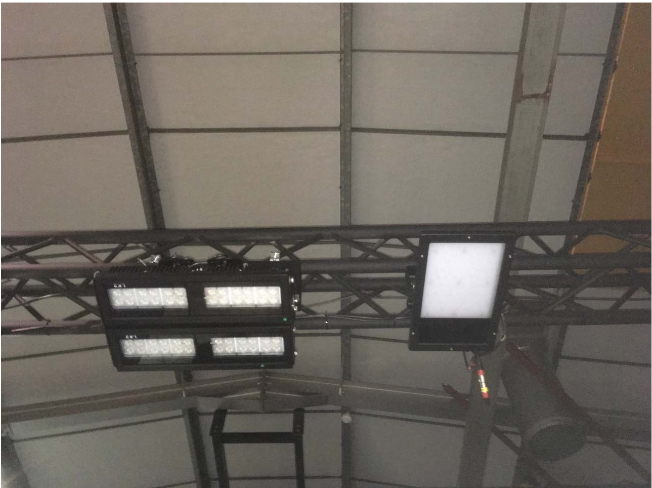
Figure 2 Lighting units at PAMELA. Left: High powered white unit; Right: Colour unit
