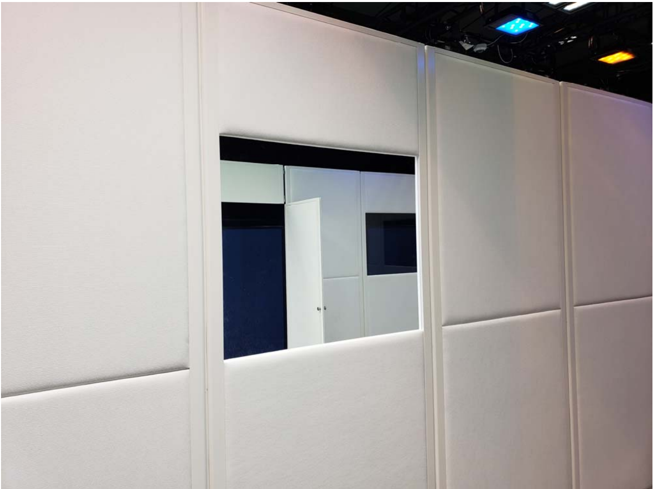
Figure 6 A prefabricated office pod used for various experiments in PAMELA. This is a commercial panel-based office unit, which can be assembled to sizes as needed using modular panel units, but is stored disassembled
